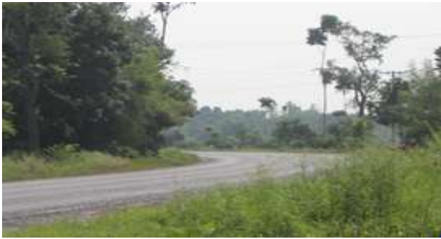
(b) Sharp horizontal curve
