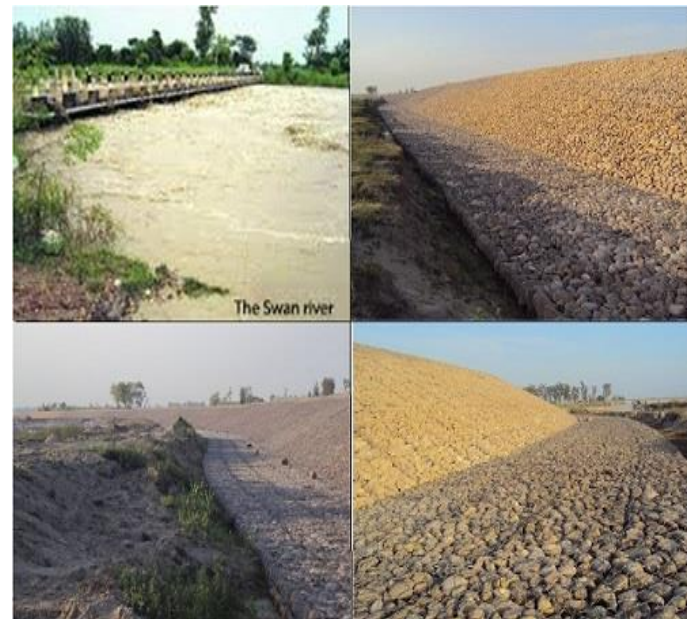
Fig. 4. Completed embankment in Phase-II
