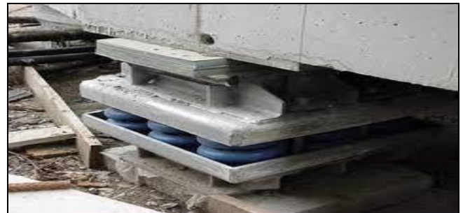
Figure 8 Spring Damper.
