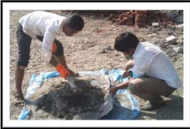
Fig 3. – Mixing of binding materials.
