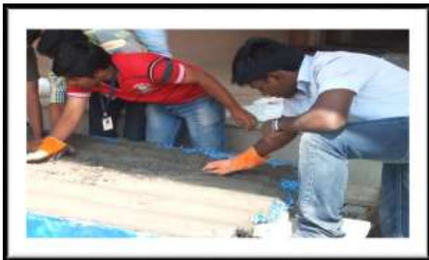
Fig 4 – Placing of Mortar.
