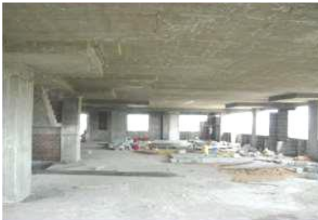
Fig. 3. Flat Slab (with drop).
