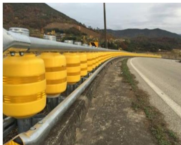
Fig. Rolling Barriers on horizontal curve
