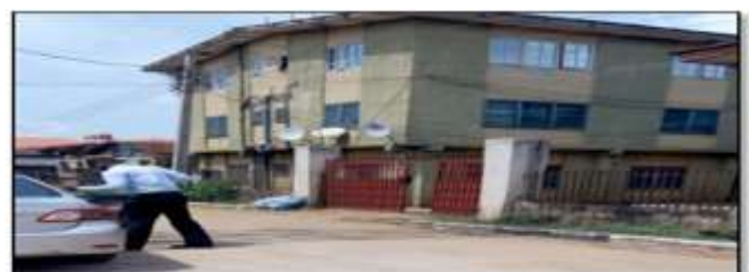
Plate 1.1: Semi-detached three bedrooms flat building, with sliding in ground floor, louvres in first floor and casement in second floor (Field work, 2022).
