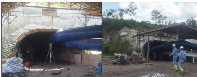
Fig. 3. South Portal of GDM underground coal mine
