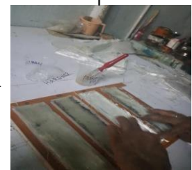
Fig 12: settling of laminate
