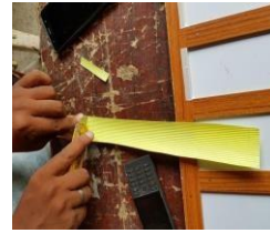
Fig 9: Applying Teflon sheet
