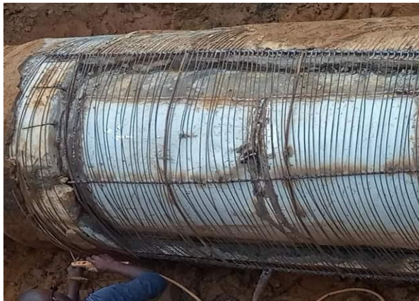
Figure 2 Repair of the 36" Transmission Main Source: Liberia Water & Sewer Corporation (LWSC)
