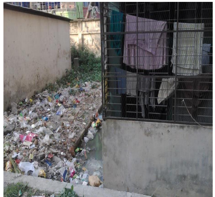
Fig. 9. Domestic wastes thrown away and drain clogging (Picture has taken from Sabujbag (Mugda))
