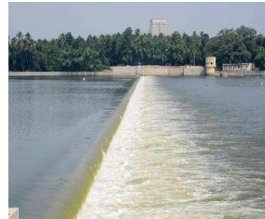
Fig. 2. Geethapuram shutter dam
