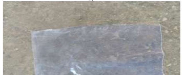
Figure .03 Liner mouth defect
