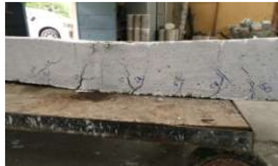
Fig. 4. Crack pattern in 40% PCA specimen
